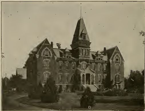
MAIN BUILDING, BOYS' INDUSTRIAL SCHOOL.
